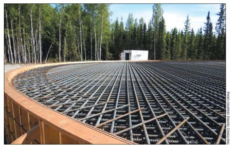
A heavily reinforced 42-inch concrete slab supports a new 70-foot-diameter water reservoir as part of the City of North Pole's expanded public water system. The design is to accommodate expected settlement of permafrost sands.
