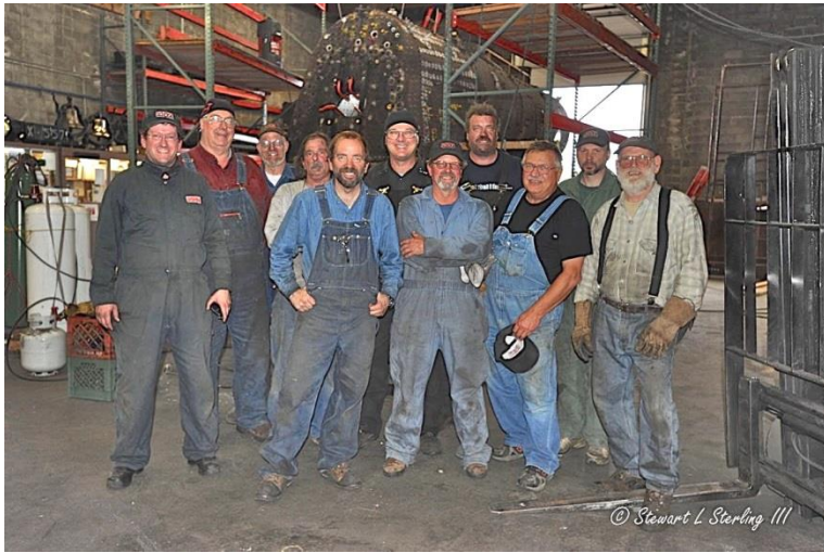
At the end of a grueling 12 hour day, all the mud ring rivets have been installed and the crew poses for a victory photo.
